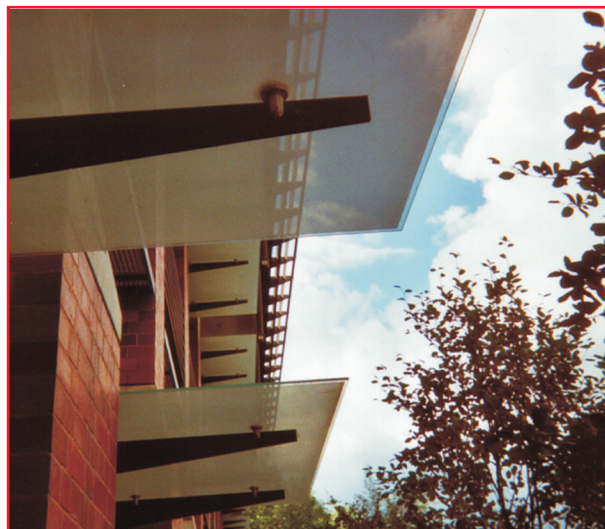
Un lightshelf (arch. Bennets Associates). 1
