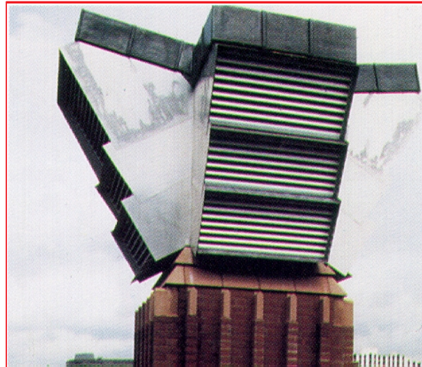
1 Cheminée d'aération, School of Engineering, Leicester (arch. Short Ford & Associates).
