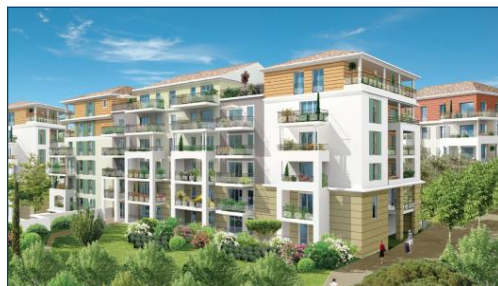
Source: doc. Bouygues Immobilier
