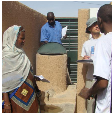
Supervision des installations
